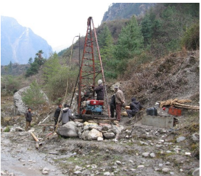
Core Drilling at Headworks Area
