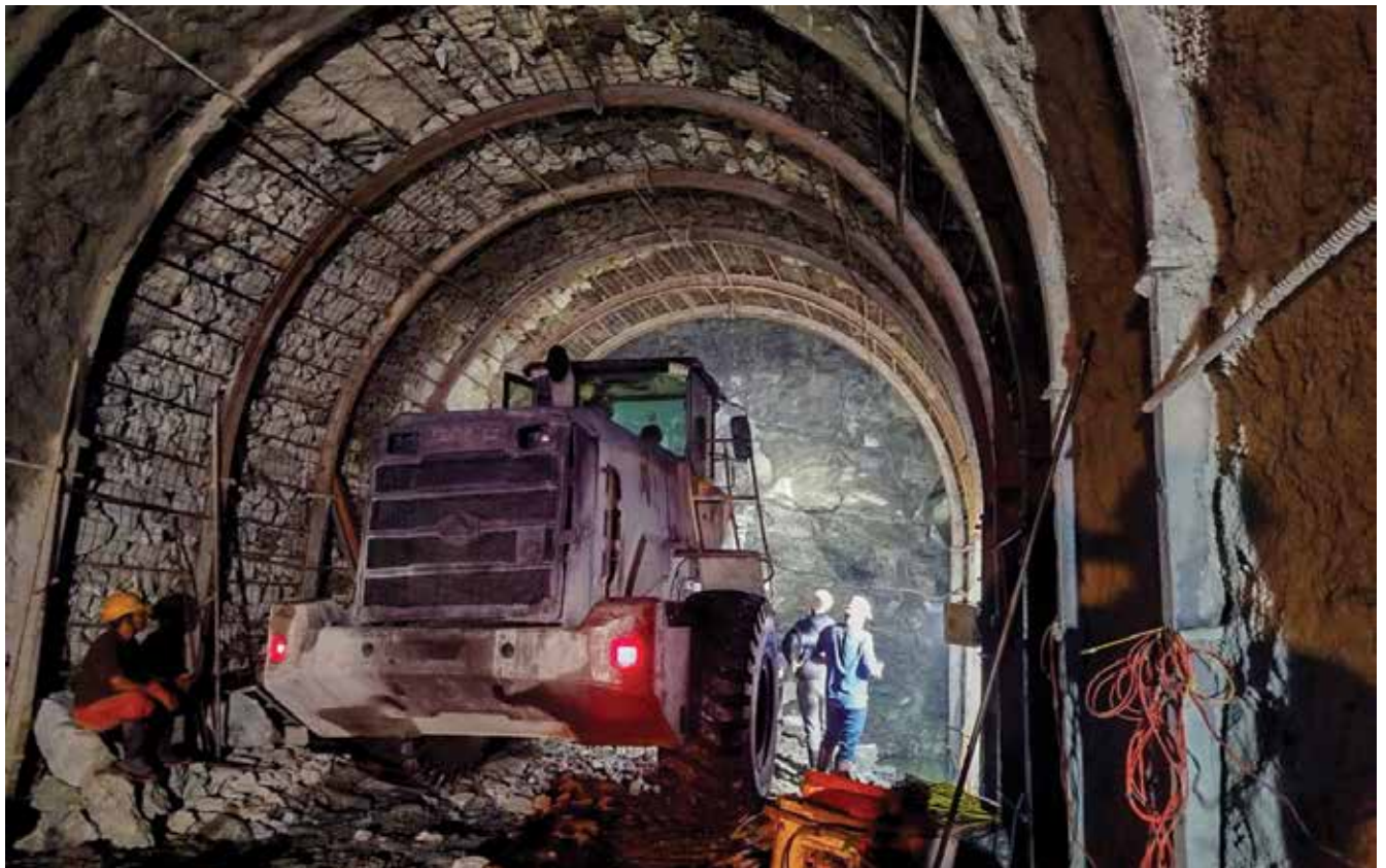
▲ Kabeli A Headrace Tunnel Excavation.
