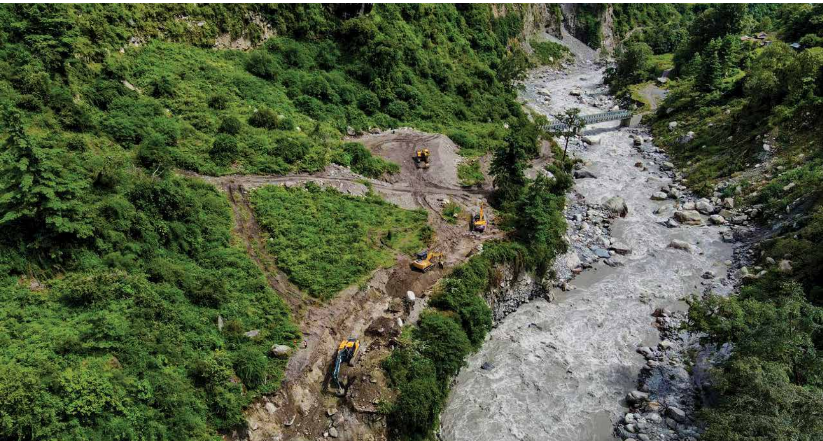
▼ MMHEP Powerhouse Area
