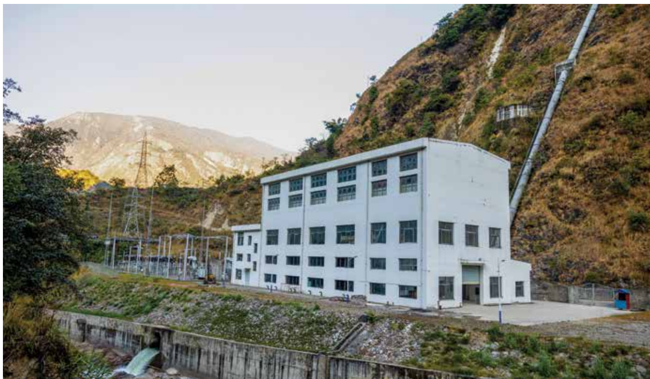
▲ Nyadi HP: Power House and Substation
