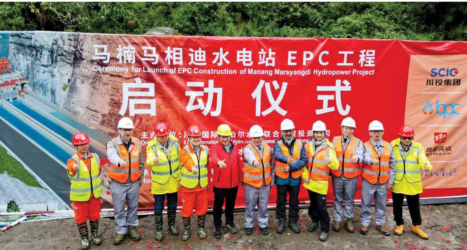
▼ Launch of Construction of 135 MW MMHEP.
